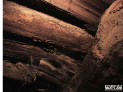
Figure 70 The Ark's decaying remains
